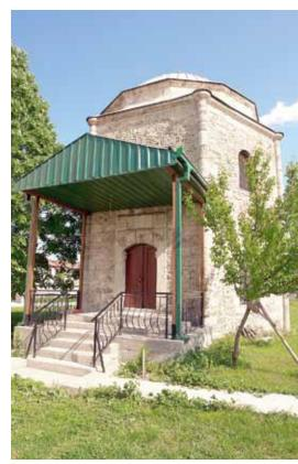
in H.1160/M.1747-48, and it was also damaged during the Bulgarian occupation in 1915 and in the earthquake of 1963. During the conservation and renovation work carried out in 1964 for the repairing of the damages caused by the earthquake, the mosque's dome was covered with tiles, the porch and part of the minaret above the serefe (minaret balcony) were reconstructed, a new mihrab, mahvil and kursī were built in the interior of the mosque, while all the interior walls were plastered.
