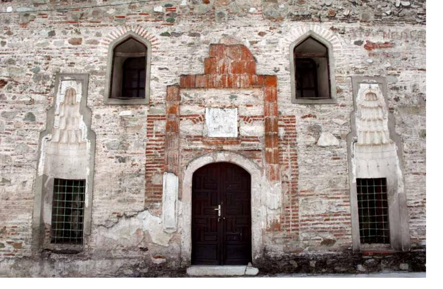
inserted bricks in some places and chiseled freestone at the corners. This opus can be seen in the small churches in the Strumica region built during the Ottoman rule in the 16th and 17th centuries.
