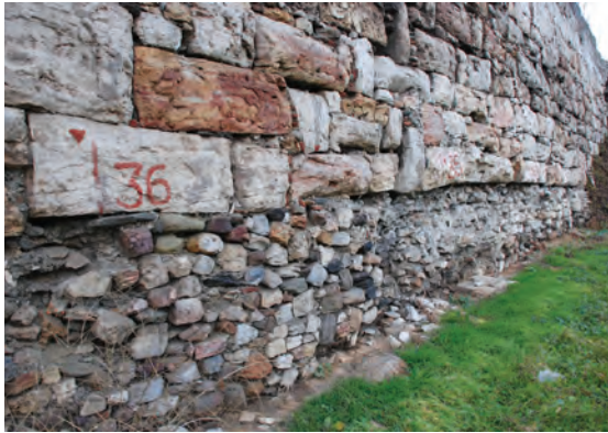
Eastern rampart section featuring both construction stages
