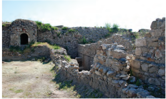
Internal partition wall of Kale VII, intercepted by the subsequent monumental Ottoman rampart
