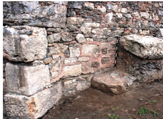
A section of the entrance to the north- eastern tower featuring the so-called cyclopean masonry and the internal side of the rampart with pink mortar joints
