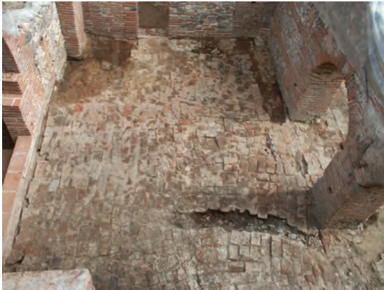
Premise no. 5, foundation
