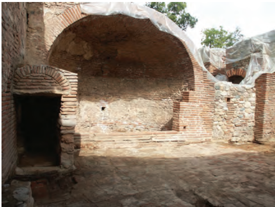
Premise no. 3, south-western wall
