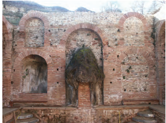
The southwest wall with two tubs and a pedestal for a fountain between them
