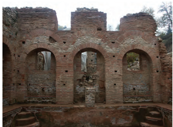
Premise no. 6, south-western wall
