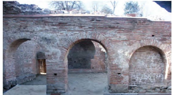
Premise no. 2, north-western wall
