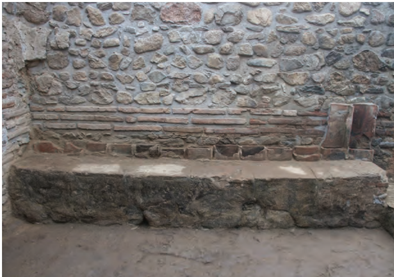
The system for heating the walls and benches of the Sudatorium
