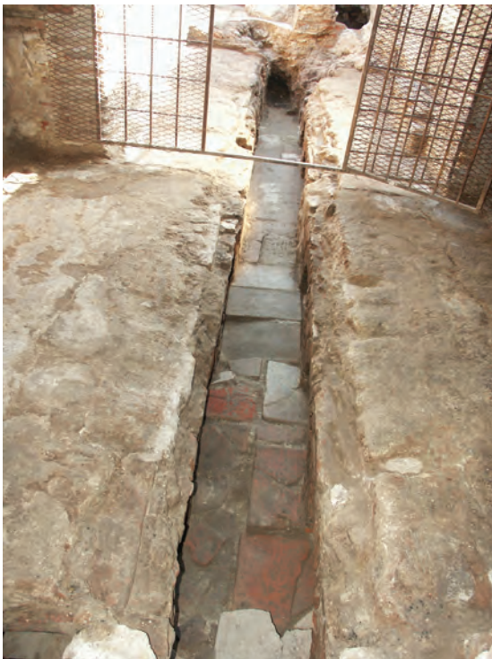
Central canal of the heating system in Premises no. 1 and no. 4
