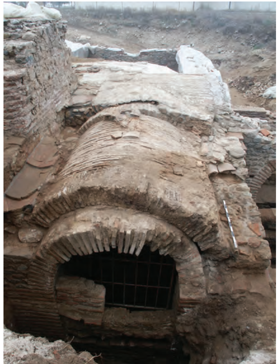
Roof construction of the Sudatorium
