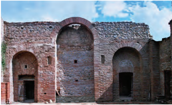
Premise No. 3, north-eastern wall
